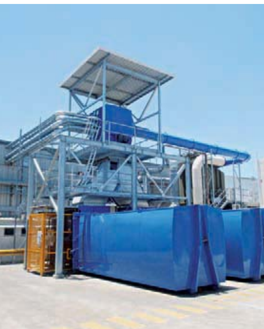
Above A new variable speed extraction system and compactor replaces the inefficient constant velocity push-pull paper waste extraction system. This has reduced electricity consumption, reduced environmental pollution from loose shredded paper, increased recycling rates and increased reliability.
